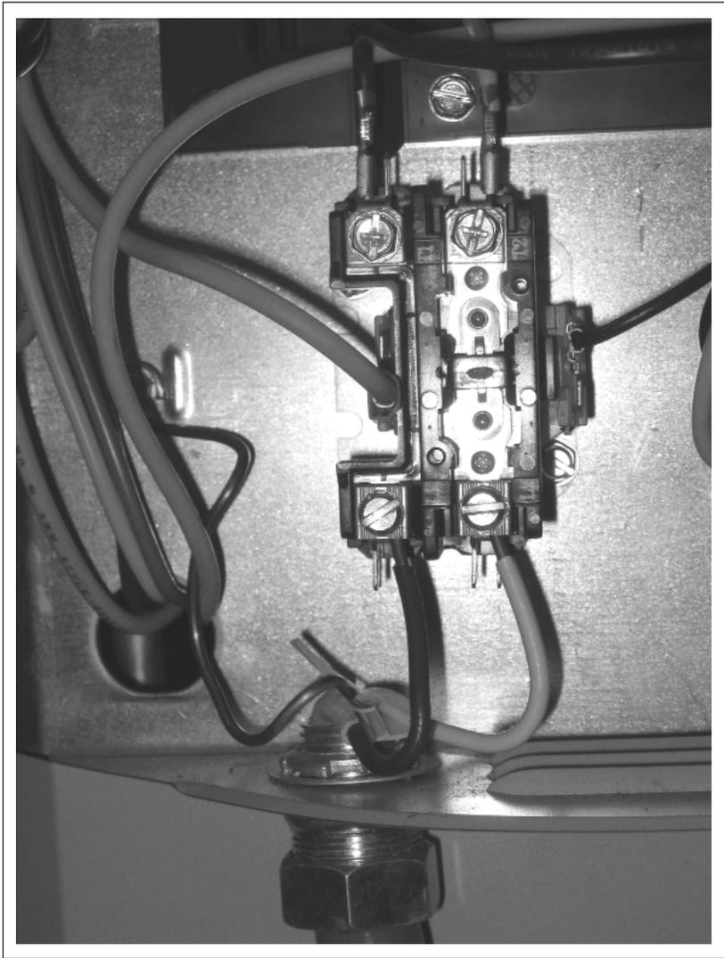
**Figure 2. Line Voltage Connections, iQ Outdoor Unit**
