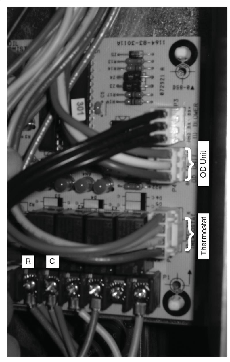
Figure 7. Control Wire Connections. Indoor iQ Interface Board.
